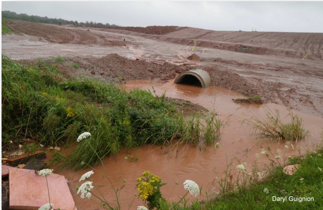
Figure 3.1 Inadequate storm water runoff control at the construction site of the new Sobeys's Mall off Malpeque Rd in 2011 during an intense rain event allowed sediment to flow directly into Hazard Creek
